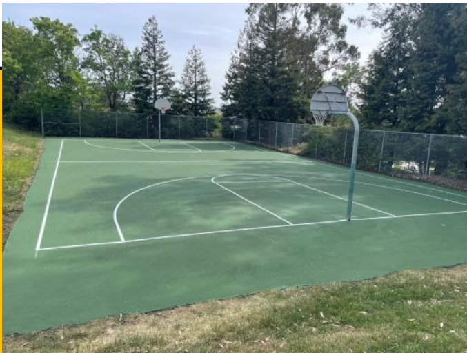
Resurfaced basketball courts at Crest Ranch Park
