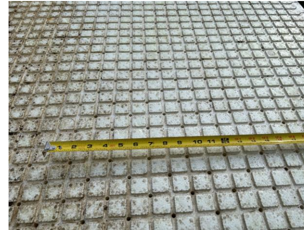
Photo #14 – Bottom side of Underlayment
