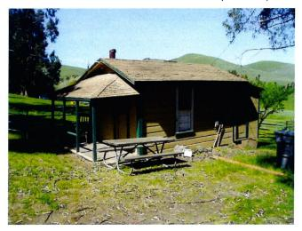
3. Tack House. A picturesque stone-walled, shake-roofed structure 20' x 42' (840 s.f.) with one large room and one small room, each with exterior entry door. The structure features a peeled timber framed veranda 10' wide running the length of the building. The veranda and building have a floor of the same stone. The timber-framed roof and porch have recently been replaced. The building is functioning as a tack room and office.
